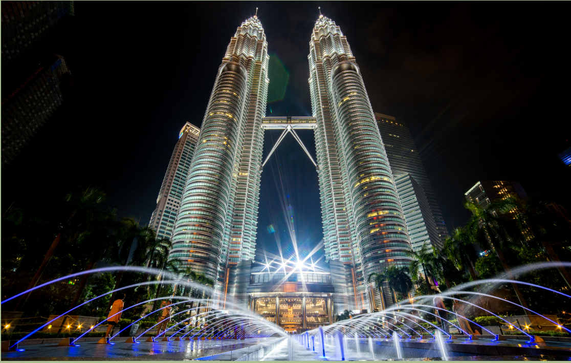
Petronas Twin Tower of Malaysia
